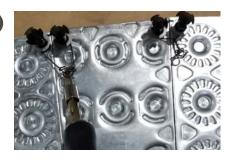
Stand on the wedge where it meets both tiles to hold in position. Tighten a rebar tie around the spacer washer on a tile and the wedge, and then the other.
