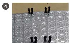
Repeat attaching rebar ties to all wedge anchors and adjoining tile anchors.
